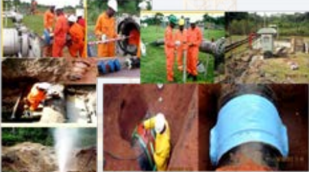
Intelligent Pigging, Cathodic Protection and On-line Leak Repairs Operation
